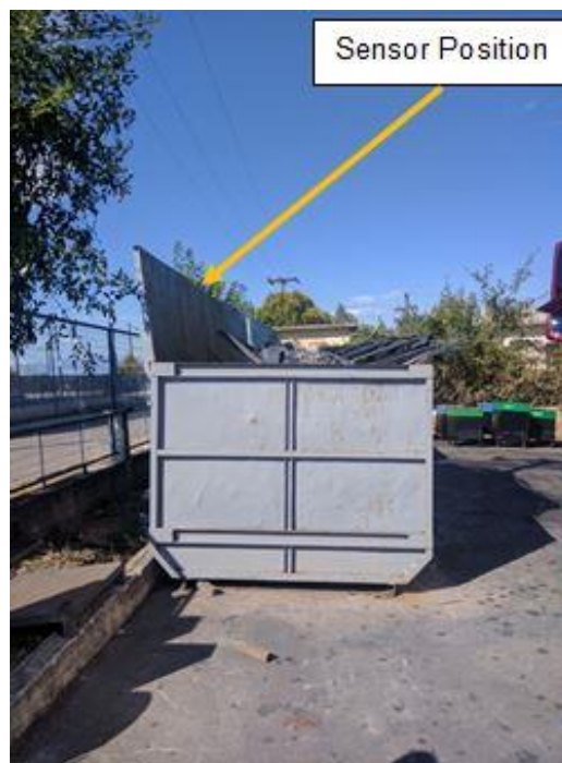
Figure 3: Fill level sensor's position
