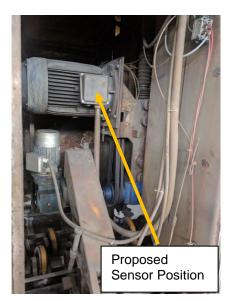
Figure 8: Proposed sensor position inside Bossi Motor
